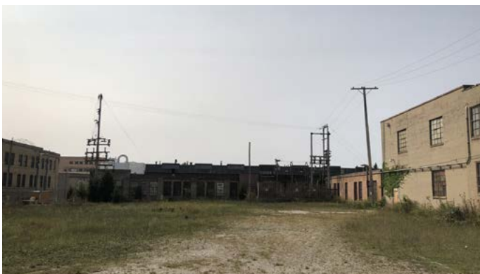
VACANT LAND AND BUILDINGS AT THE 30TH STREET CORRIDOR BID
